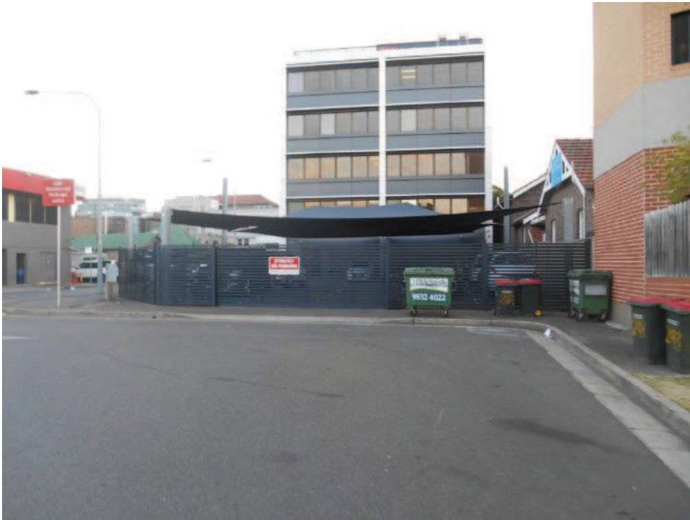
View of Building at 10 Phillip Street, from Lennox Bridge Car Park
