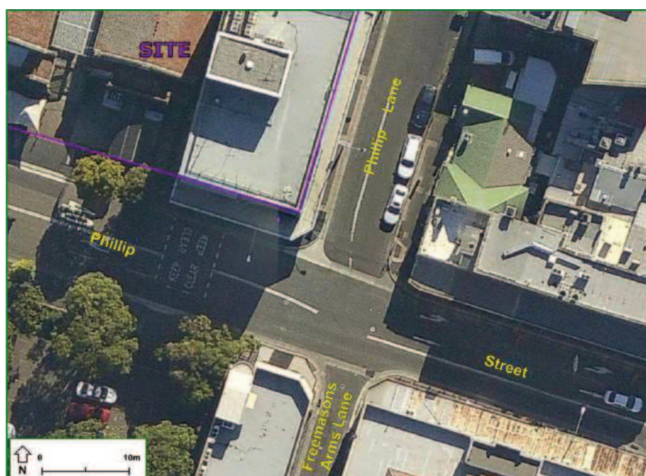
Figure 5: Phillip Street / Freemasons Arms Lane Intersection
